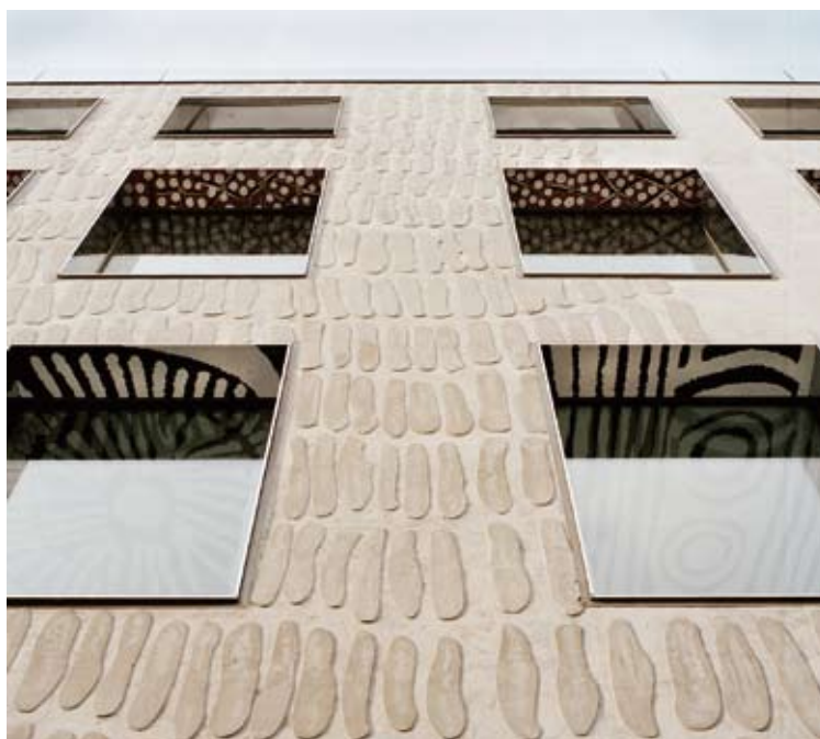
Facade of the administrative building featuring Jimbala and Kumerra , by Aboriginal artist Lena Nyadbi, 2005 photograph by Antonin Borgeaud Musée du quai Branly
