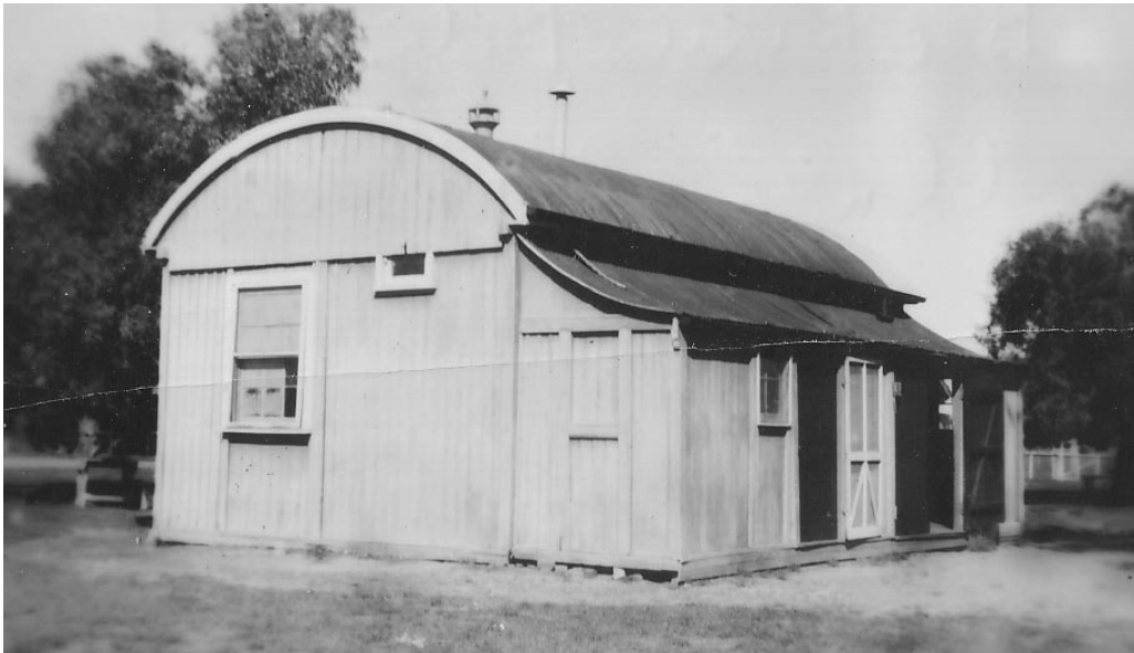
Inspector Mitchell's photograph of the beehive school building at Pallamallawa, around 1950 courtesy UNERA, HRCF collection, 1374
