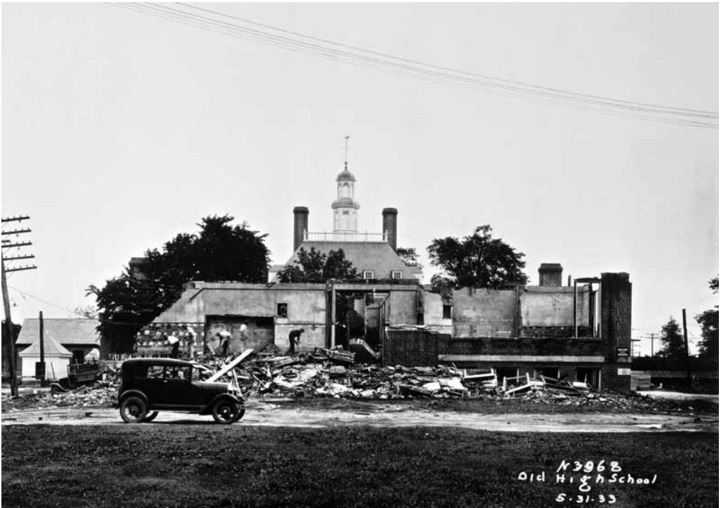
Figure 7. Demolition of Matthew Whaley School, Williamsburg, Virginia, to make way for the reconstructed Governor's Palace, early 1930s
